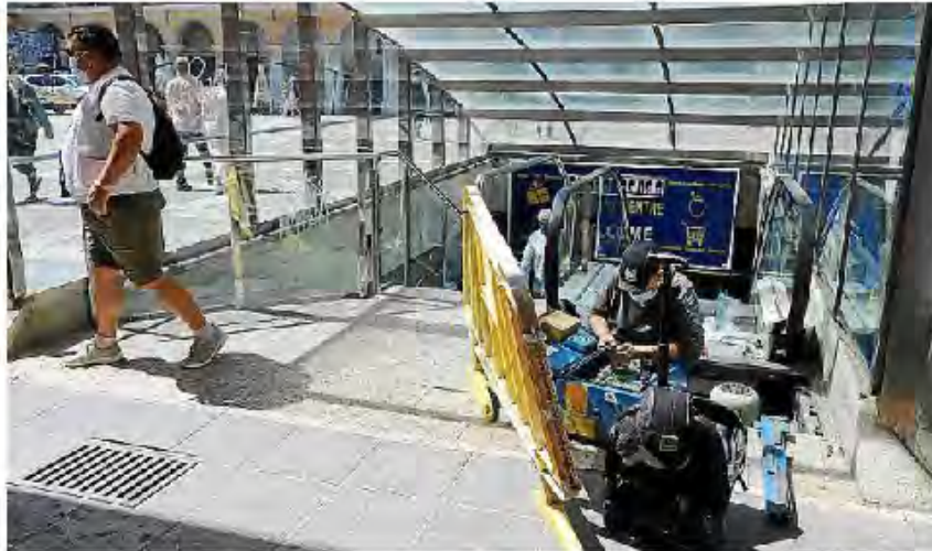
Repairing the escalators. 12-05-2021 Teresa Ayuga
